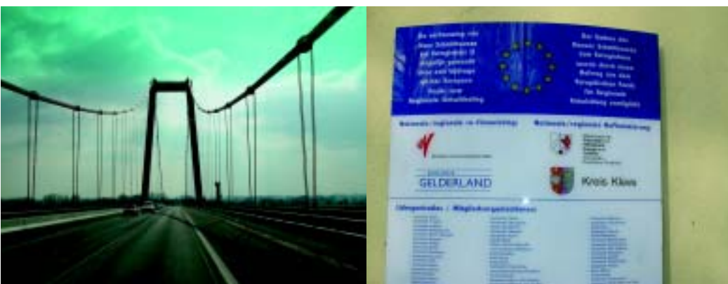
Left: Rhine bridge at Emmerich (Germany).
