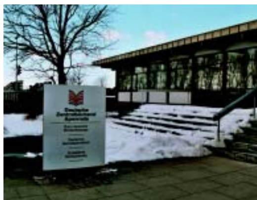
German central library and office of the Association of Germans in North Schleswig in Aabenraa (ge. Apenrade).
